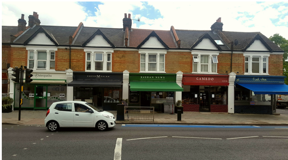
High Street Colliers Wood: Before and after
